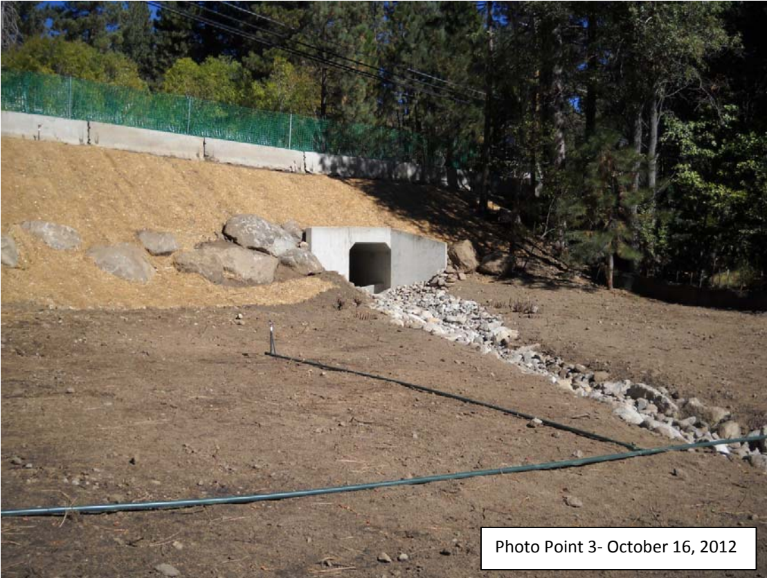
Photo Point 3 – downstream end of new culvert at Northwood Blvd
