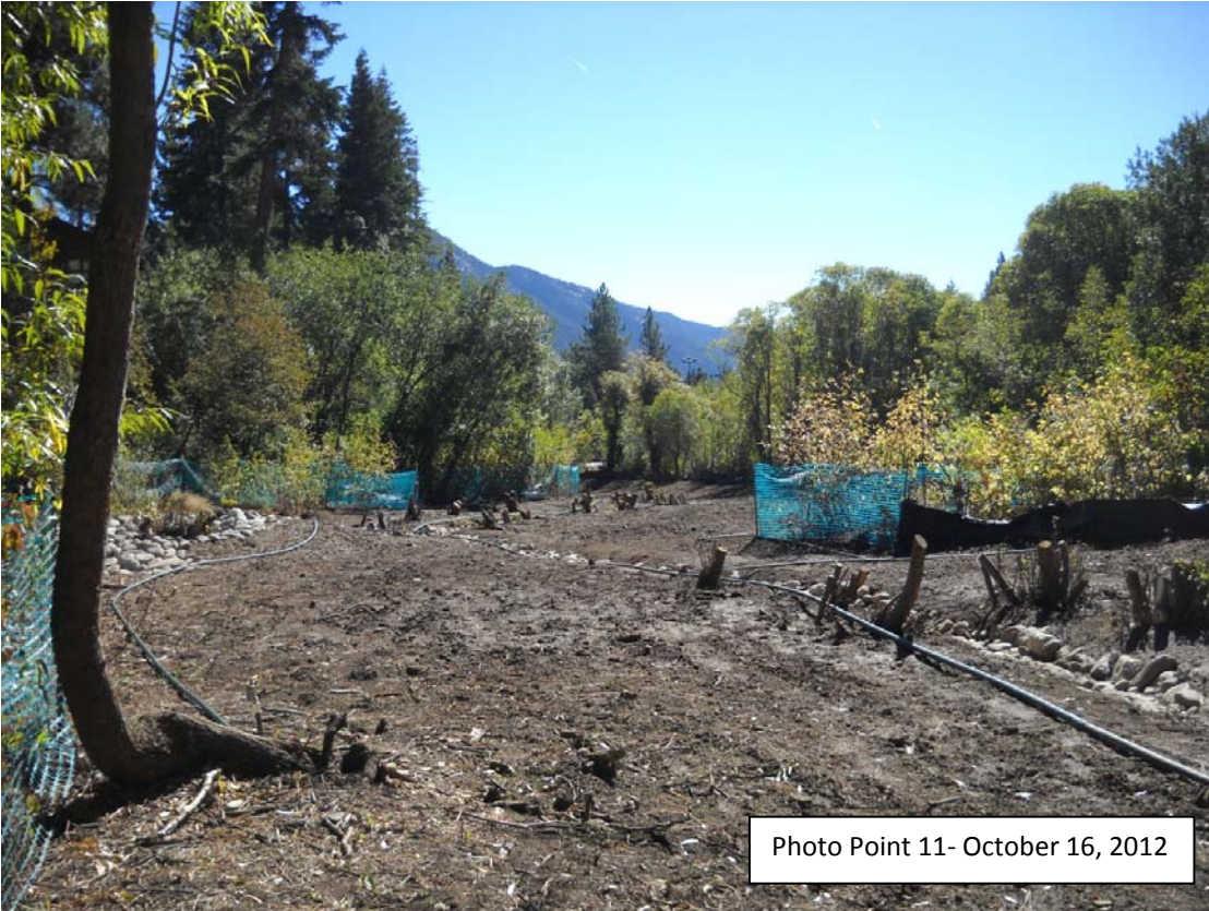
Photo Point 11 – Floodplain and willows clumps looking downstream on new channel
